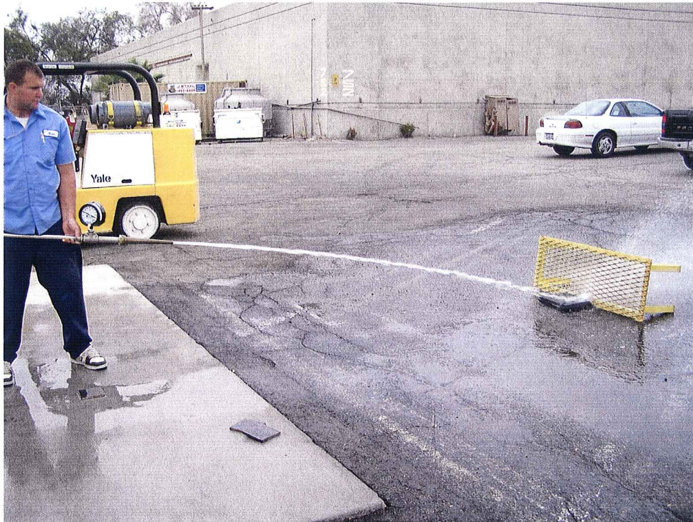
Photograph 3 Rain Intrusion Test Setup
